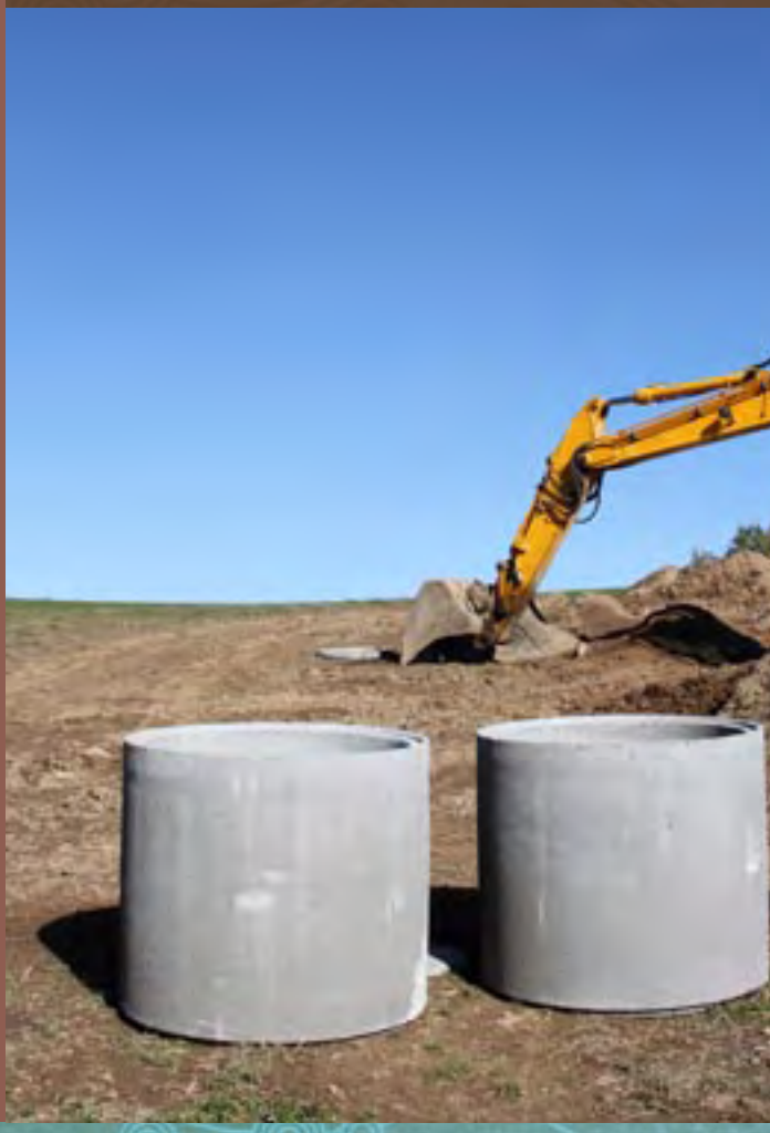
▼ Concrete pipe segments at construction site.
