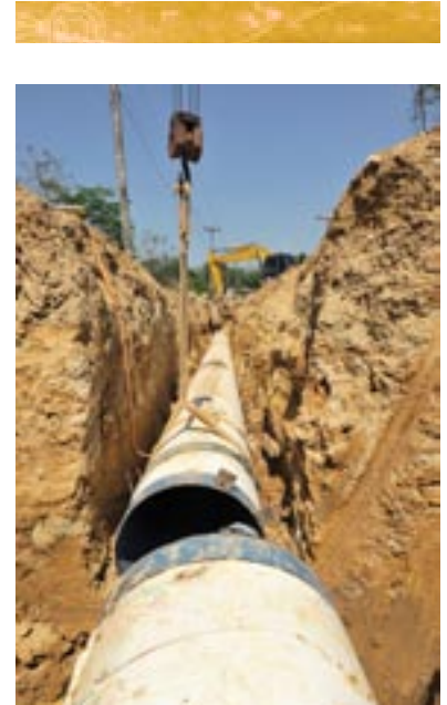
Laying water pipes in a construction area.
