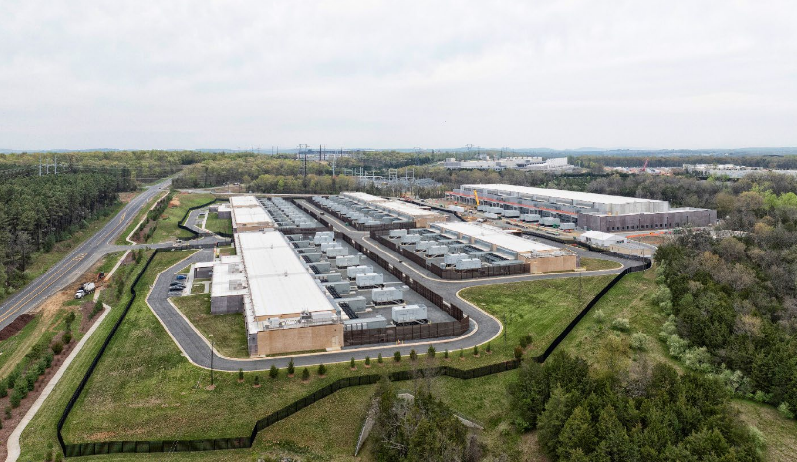
A data center in Leesburg, Virginia.
