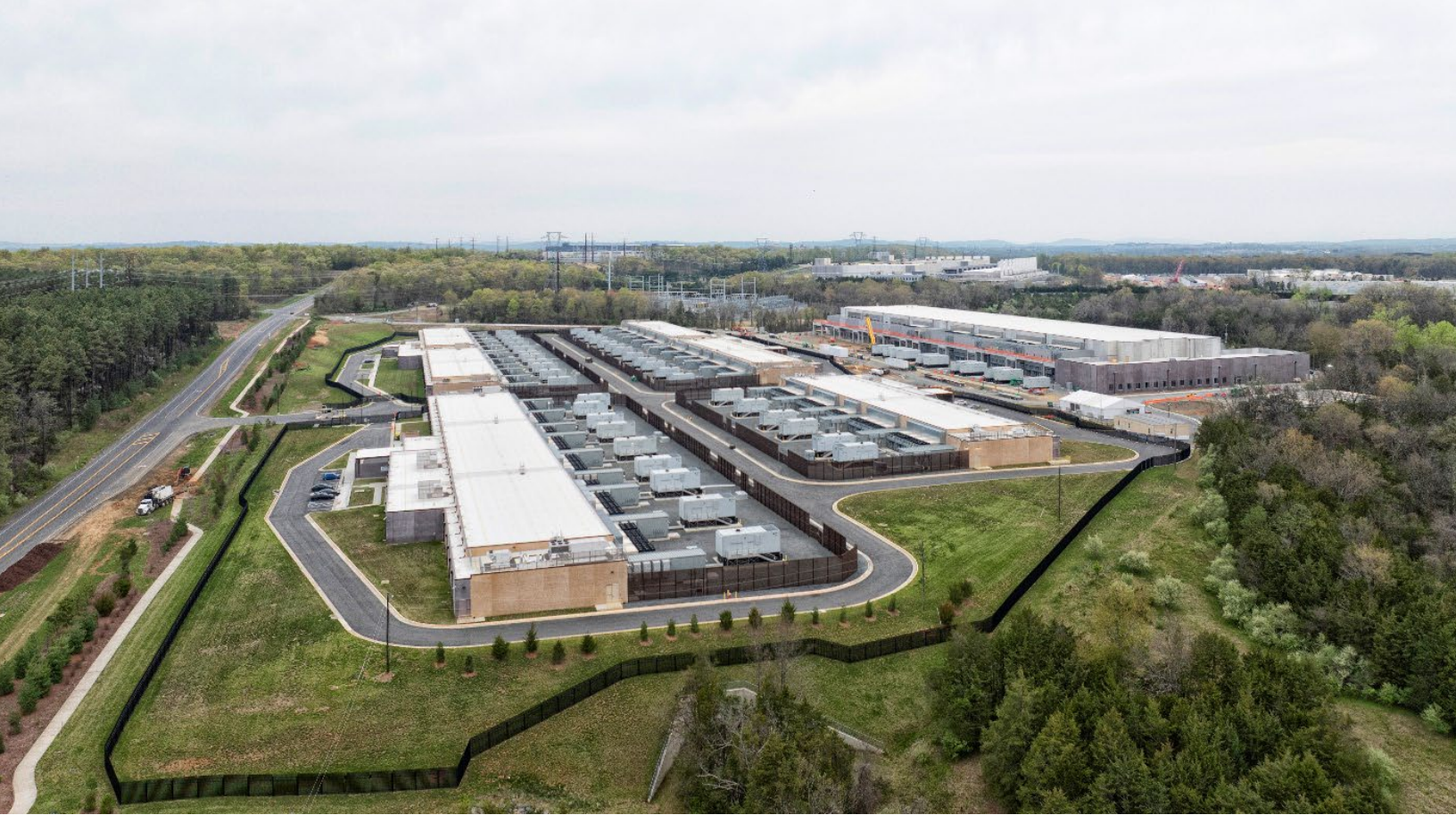
A data center in Leesburg, Virginia.
