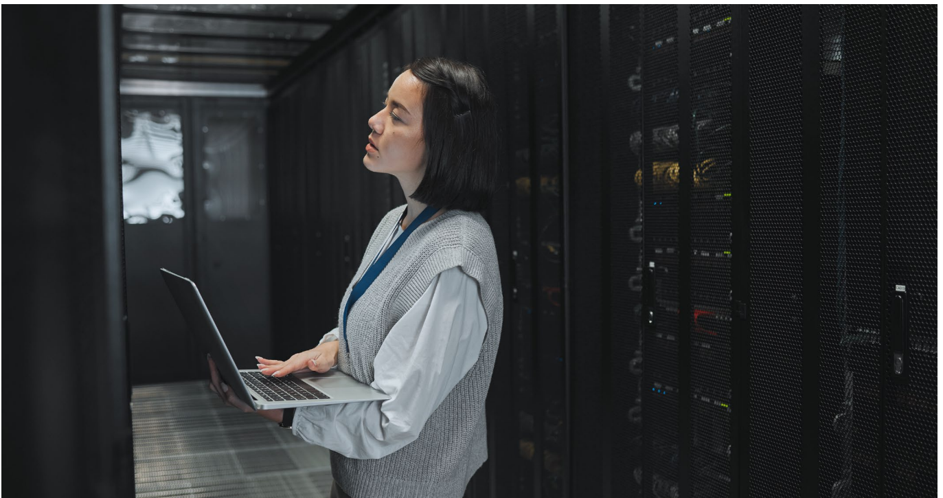
A person works inside a data center.
