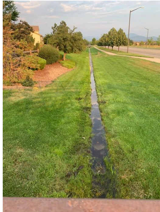
The trickle channel lined with Kentucky bluegrass before the Black Bird Knolls conversion. (Photo credit: Black Bird Knolls HOA).
