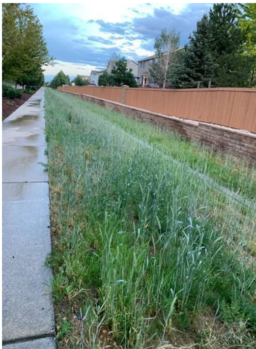
The trickle channel after the conversion, with newly planted and still growing native grasses (Photo credit: Black Bird Knolls HOA).
