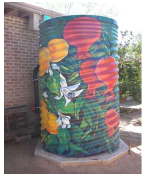
Rainwater harvesting tank. Photo: Christina Bickelmann
